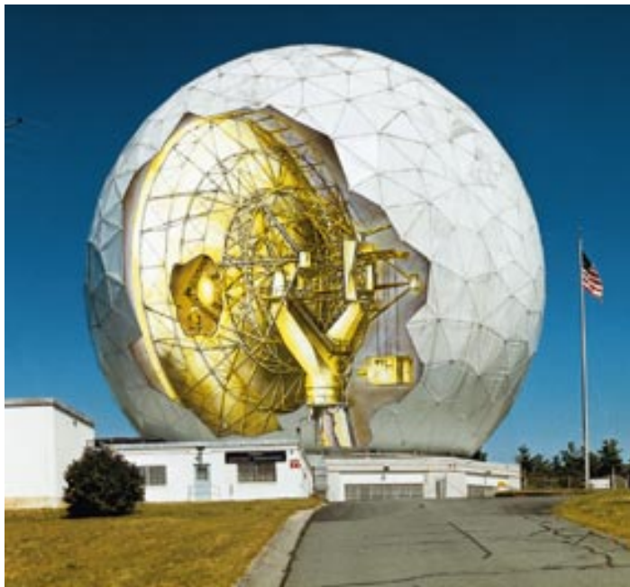
A cutaway view of the Haystack antenna showing the Cassegrain subreflector and the hoisting system for the interchangeable equipment boxes.
