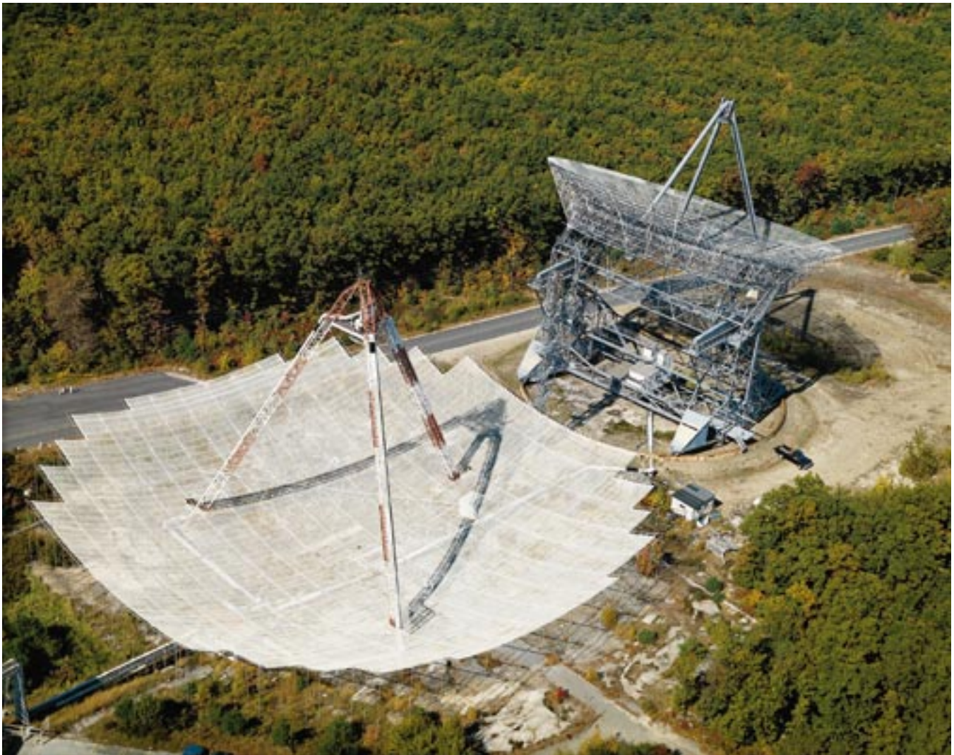
Millstone Hill incoherent scatter radars use a 68-m zenith-directed dish and a 46-m fully steerable antenna.
