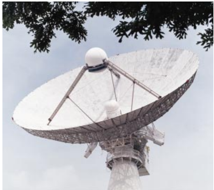
The 26-m diameter antenna of the Millstone Hill L-band satellite tracking radar.
